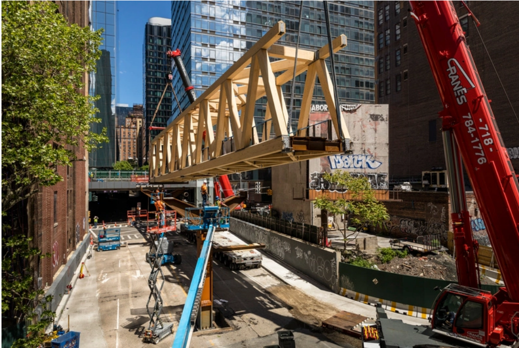
The installation of the new Timber Bridge, connecting the High Line Spur's Woodland Bridge to Manhattan West and Moynihan Station. Photo by Andrew Frasz, courtesy of the High Line, New York.
